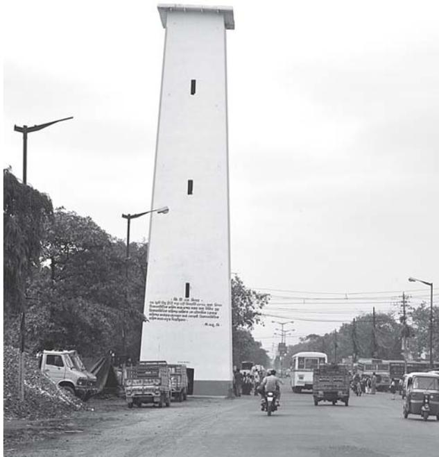
Trigonometric Survey tower on B.T. Road, Kolkata. The inscription says, "G.T.S. Tower. This 75-ft brick tower was built in 1831 for the Great Trigonometric Survey conducted by George Everest, Superintendent of Great Trigonometric Survey and Surveyor General in charge of all topographical & revenue surveys."
